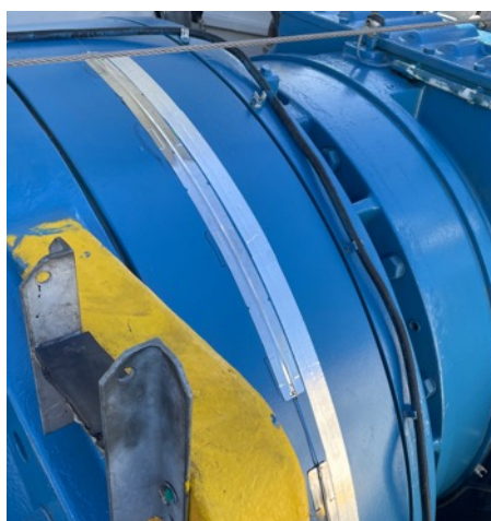
Figure 3: Example GearUp strip installation up-tower
